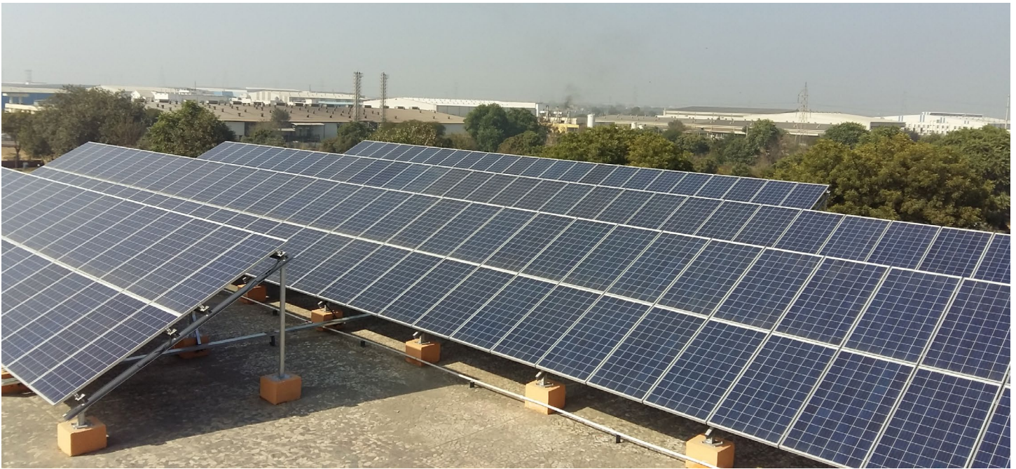
Solar panels installation at our Bawal, India facility.
