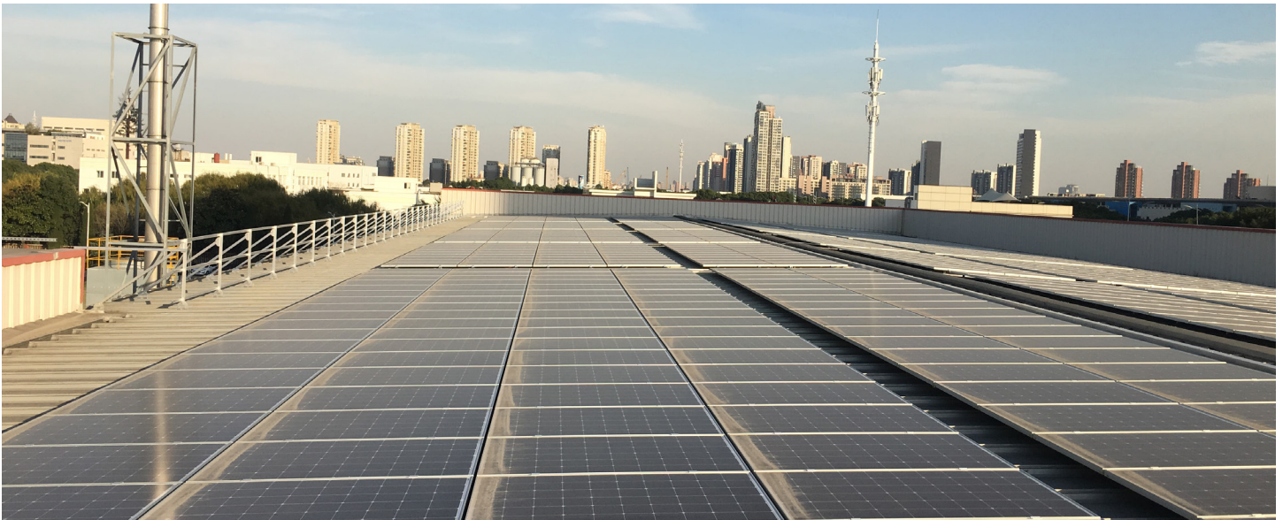
Solar panel installation in Suzhou, China.
